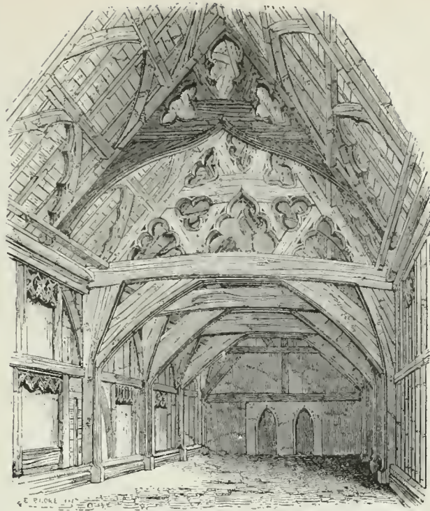
ROOF: WITH CAMBERED CROSS BEAMS CARRYING A DECORATIVE SYSTEM OF BRACES AND STRUTS.
